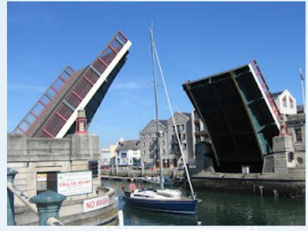
The works mainly involve the repair of the steel deck plates and steel sections which support them. Other works include the painting of the elevations and parapets, stone cleaning and repair of the lanterns.
