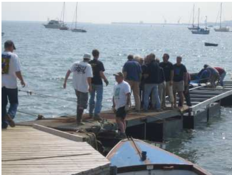
Getting the pontoons into position - Richard White
