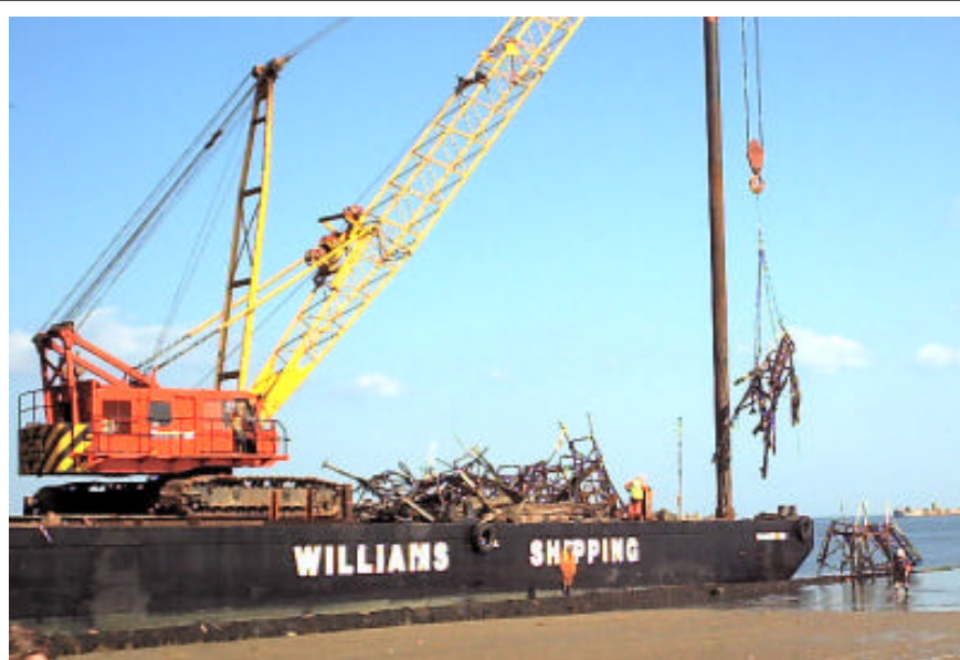
The last remnants of the pier being removed
